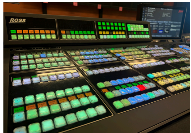
Ross Video Production switcher
